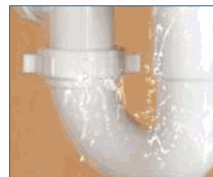
Pipeline cracks and water leakage
