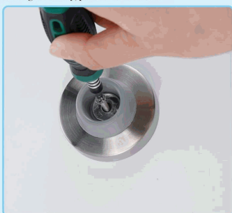
Step 4: Install screws to fix the door stop.
