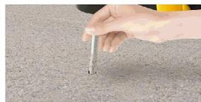
**Step3** Tap the anchor screw into the hole.
