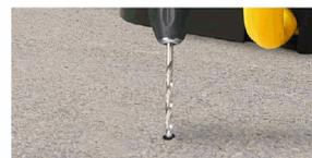
**Step2** Use an electric drill to drill a hole.
