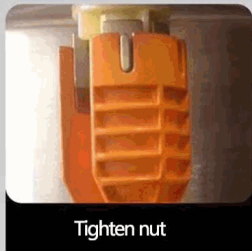
Tighten the pipe joint
