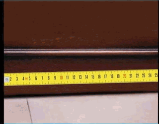
Measure the width door or window
