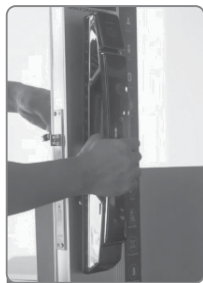
5 Mounting front panel
