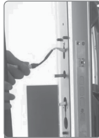
11 Connect the rear panel data cable
