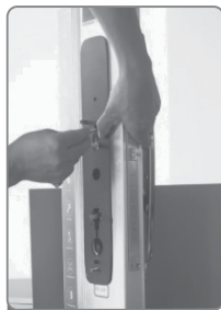
6 Secure the rear backplane plate
