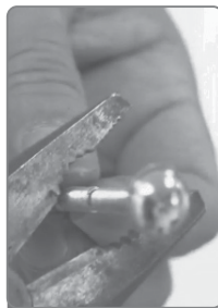
7 Cut screws according to doorthickness
