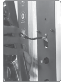
12 Data cable into the door hole
