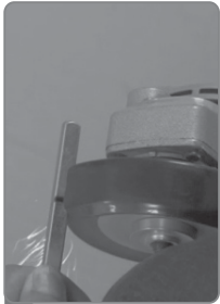
9 Cut excess square steel
