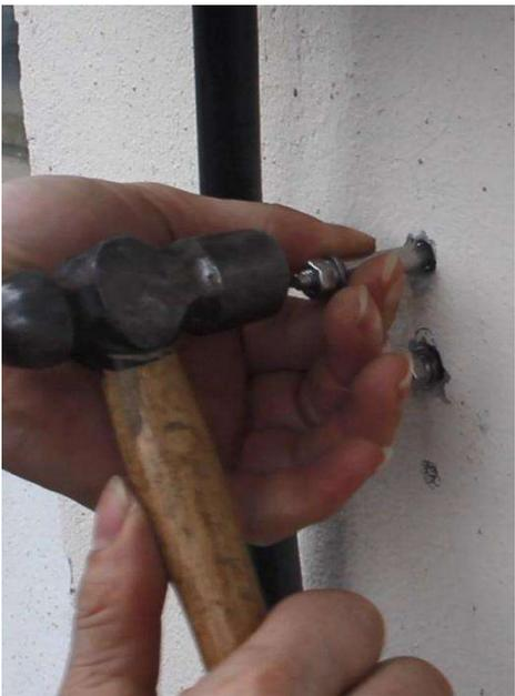
11. Drive the expansion screws in with a hammer.
